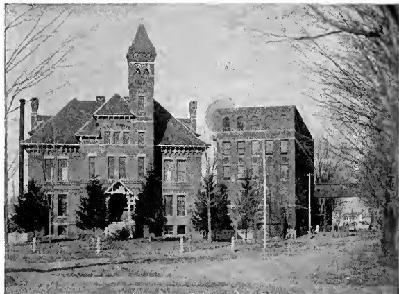
A Chicopee Falls School Building
